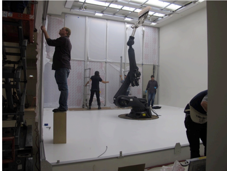
Fig. 19 Installation of barriers around the robot enclosure
