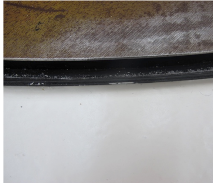
Fig. 16 Gasketing installed around the robot's circular mount to prevent seepage of liquid under the decking
