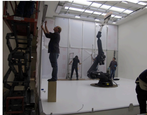
Fig. 6 Image of polycarbonate barrier, as being installed
