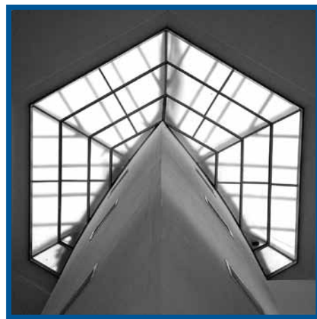
small rotunda skylight
